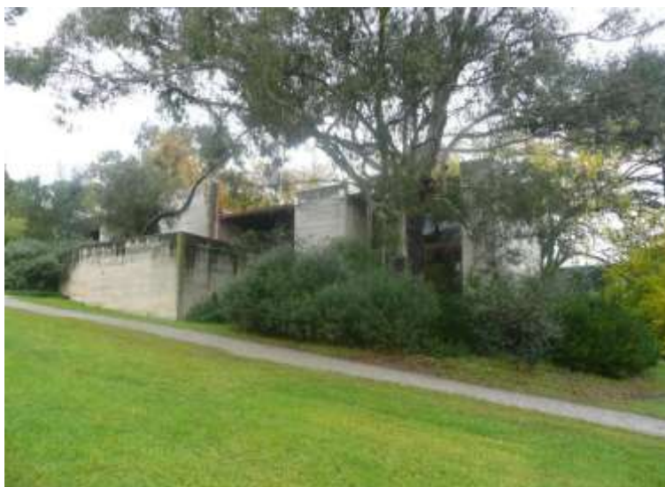
Heide II (Reed house, Bulleen, 1967) Heide Museum of Modern Art, Melbourne Architect: David McGlashan
