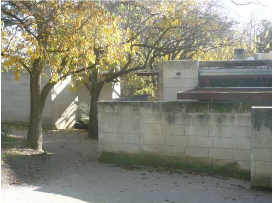
Heide II (Reed house, Bulleen, 1967) Heide Museum of Modern Art, Melbourne Architect: David McGlashan, McGlashan Everist Pty Ltd Architects
